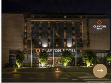
Clayton Hotel Leopardstown DUBLIN, IRELAND 357 rooms
