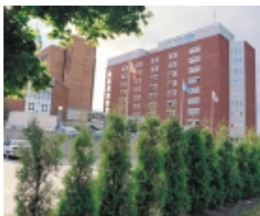
Quality Hotel Nacka, 146 rooms Southern Stockholm
