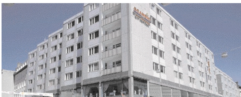
Scandic Hotel S:t Jörgen, 265 rooms Central Malmö
