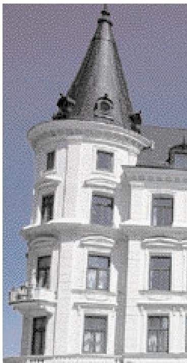
Provobis Hotel Kramer, 113 rooms Central Malmö
