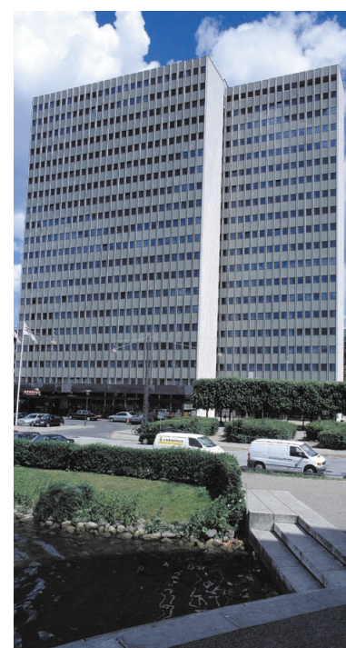
Scandic Hotel Copenhagen, 470 rooms Central Copenhagen
